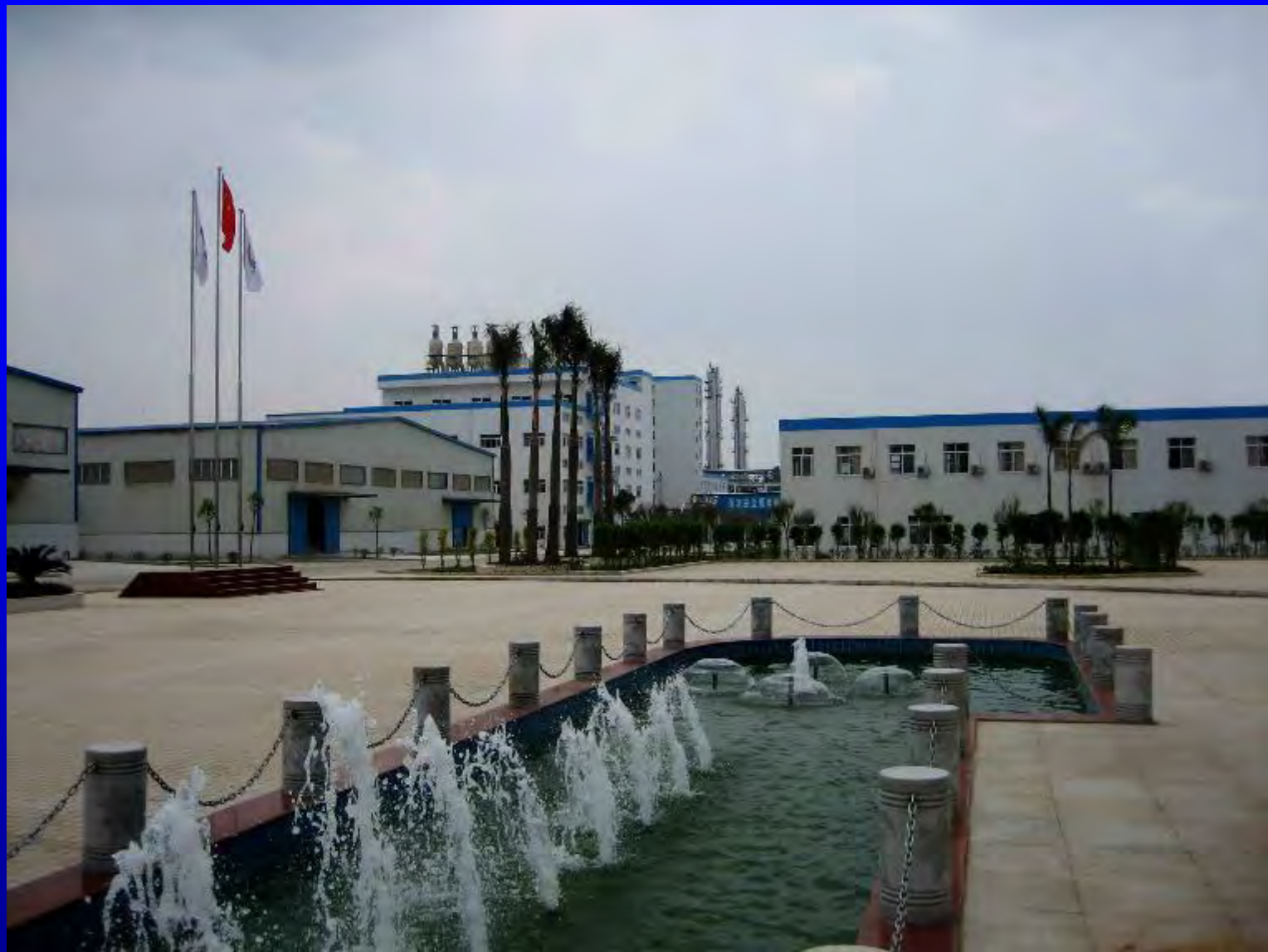
COFCO cassava-based ethanol factory in Hepu, Guangxi, China, with a capacity to produce 840,000 l ethanol/day, requiring about 4,500-5,000 tonnes fresh roots/day
