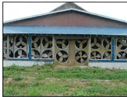
↑牛舎壁面の換気扇
