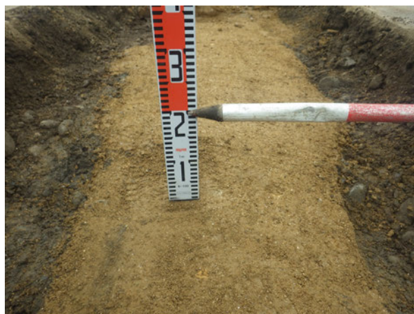
掘削深さ確認 (H=0.2m)
