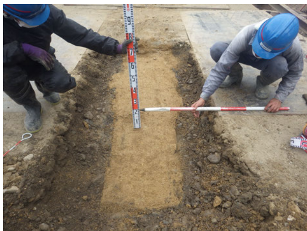
掘削深さ確認 (H=0.2m)
