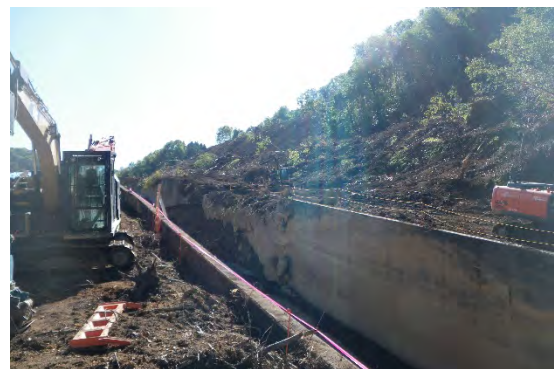
[洪水吐急流水路付近]
