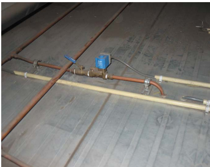
Fig. 6.14.1.3 Secondary solenoid valve controlling entry to a store room
