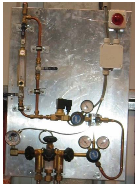
Fig. 6.14.1.2 – Ethylene station and cylinders
