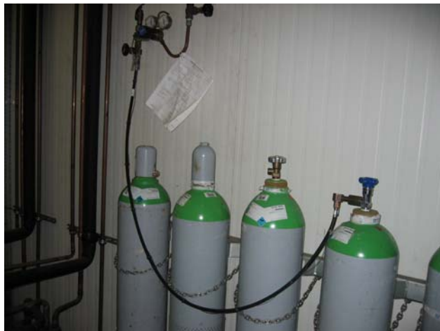
Fig. 6.14.1.2 – Ethylene station and cylinders
