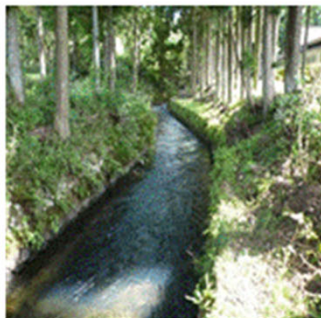
Masonry canal with pure flowing water
