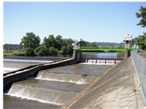
Head work installed on the left bank of the Karasugawa which is the water source
