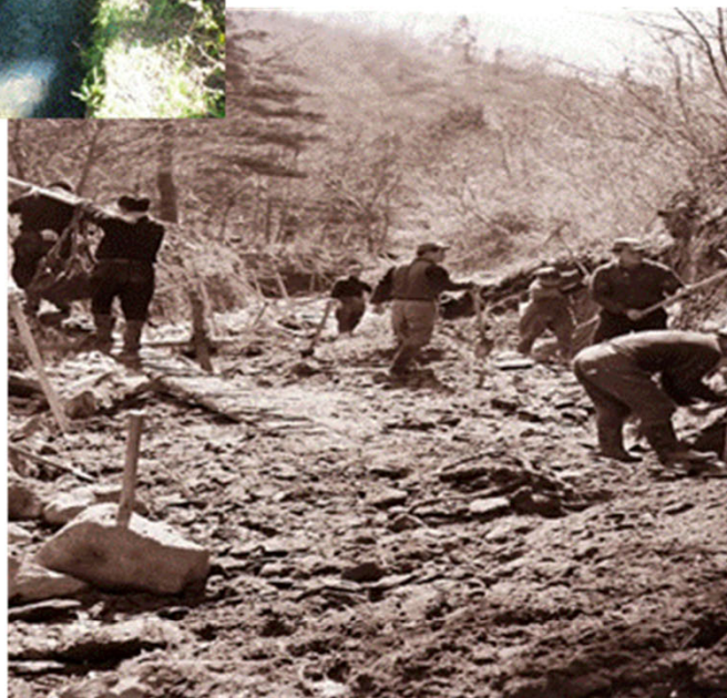
Canal repair work in 1954
