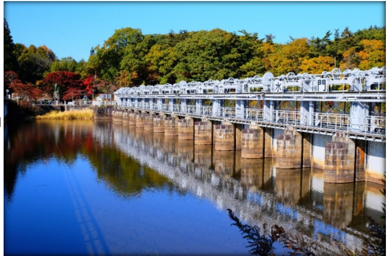
Current Jurokkyo Sluice Gate
