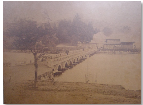
Former Jurokkyo Sluice Gate
