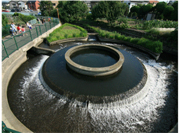
A cylindrical diversion weir installed in 1962
