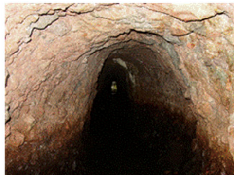
Lake Haruna Tunnel completed in 1904
