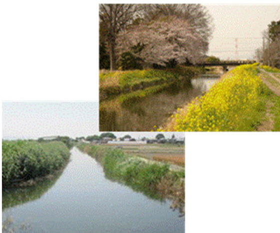
Canal section excavated without timbering that conveys the vestiges of excavation to date
