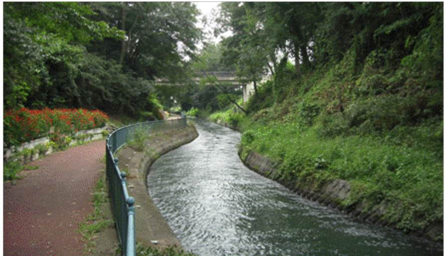
"Tenguiwa irrigation canal" excavated by Lord Akimoto Nagatomo
