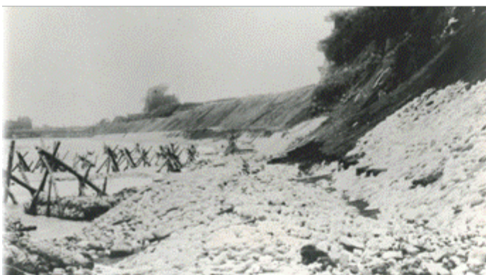
The "etchu-waku" groyne construction method been used near the Tenguiwa intake since times of yore
