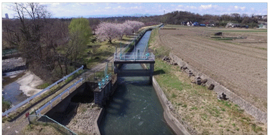
The "sluice gate" and "spillway gate" renovated in the irrigation drainage project in 1998
