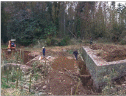
Excavation of the former intake gutter gate
