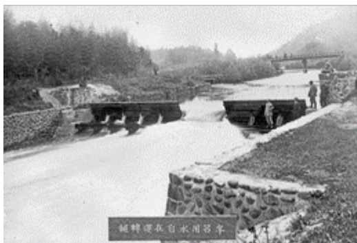
Free-operational gutter (Muro irrigation)
