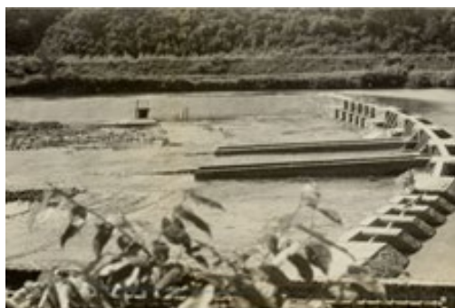
Weir made of artificial stones
