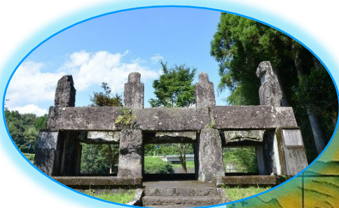
Hyakutaroumizo / Former intake sluice
