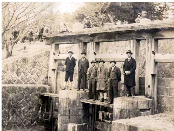
Gutter gate and irrigation managers
