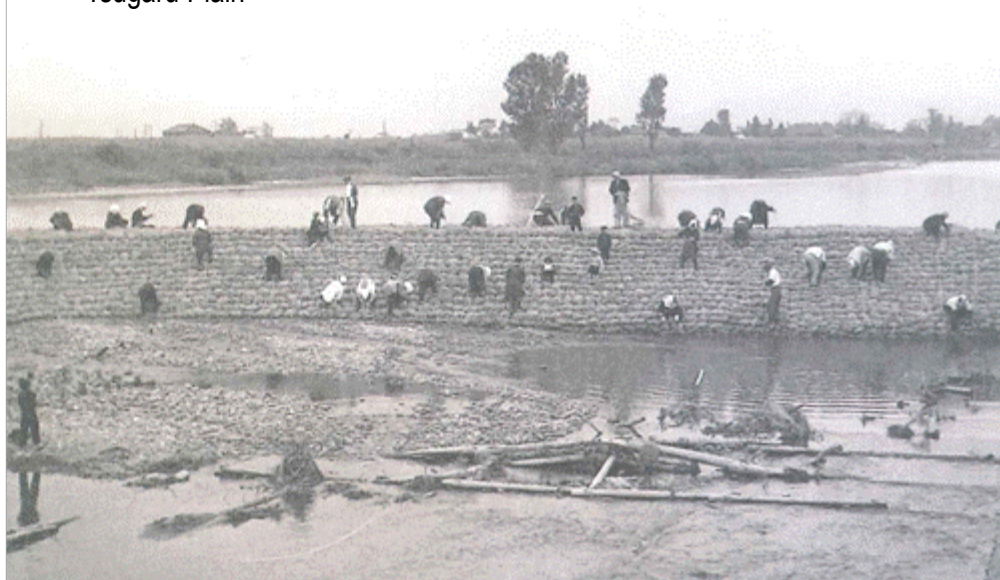
Doen weir repair work pre-1958 (heaping up bales)
