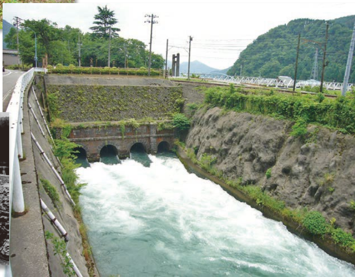
Current water inlet
