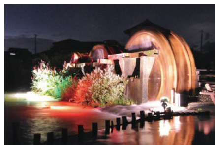
Asakura triple water turbines (illuminated)
