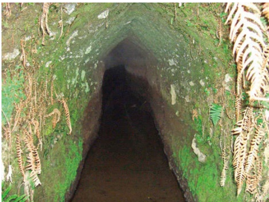
Inside the waterway tunnel
