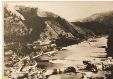
Tachibai weir in around 1907
