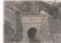
Yamadagawasosui No. 2 Tunnel
