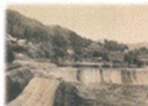
Water source stone dam of the Ougogawasosui
