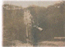
Iwaoka branch line Steel pipe siphon, Yamadagawasosui
