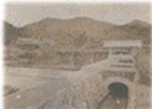
Full view of Yamadagawasosui water source dam
