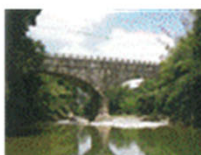
Misaka Siphon (two-arched bridge)
