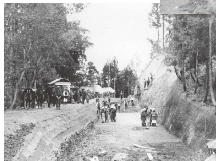
Uwaeyousui irrigation canal repair work at Yonemasu in 1915
