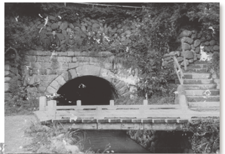
Kawakami tunnel in around 1931
