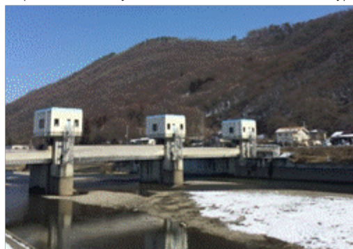
Jikkasegi head work that takes water from the Narai River
