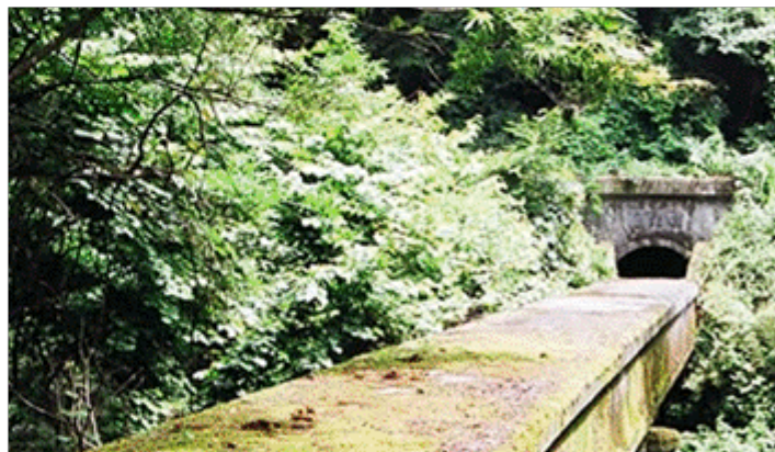
Waterway bridge (Source: National Midori Net "Agricultural Waterway Directory HP")
