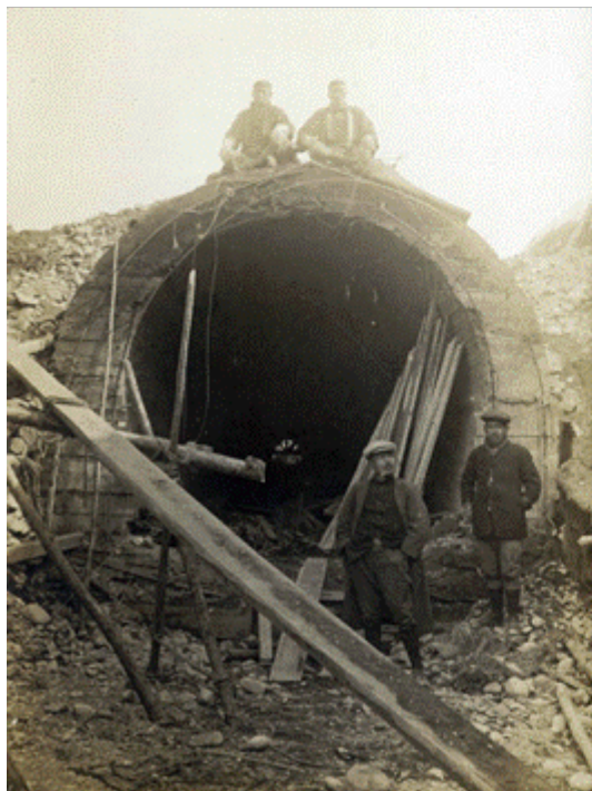
Photograph of the time when the river crossing was renovated from a plane crossing to a siphon (Taisho 9th year, 1920)
