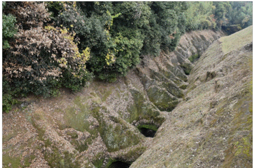
"Hanaguri Ide" (Baba Kusunoide canal) that functions to suppress sediment accumulation
