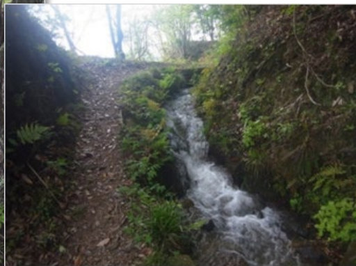
Energy dissipation work utilizing the natural terrain (granite)
