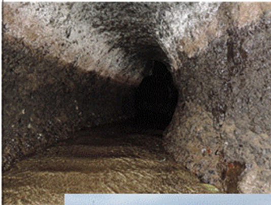
Inside the Hoi Tunnel
