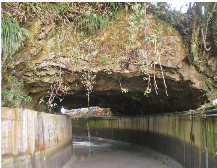
Traces of rock excavation
