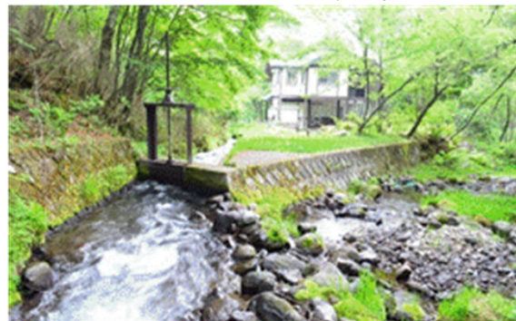
Shibatatae (Ohkawara-segi Intake), with a structure that intentionally leaks to secure downstream water as required
