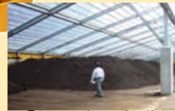
Compost production facilities
