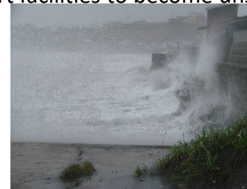
Wave overtopping by high waves
