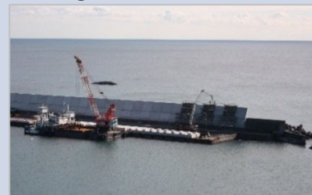
Raising of breakwaters
