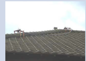
Sprinkler installation on barn roof
