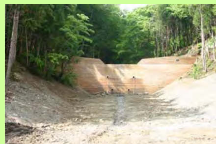
Erosion control dam
