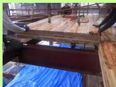
CLT floor structure installed onto high-rise building (Saga)
