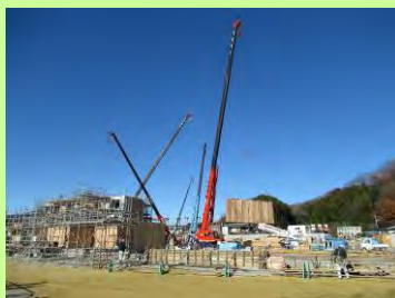
Installation of CLT panels (Fukushima)
