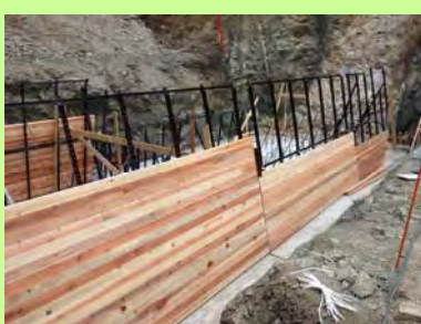
Wooden remaining formwork
