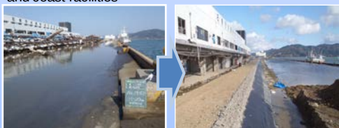
Ground subsidence of a fishing port caused by the tsunami and the status of reconstruction through raising embankments
