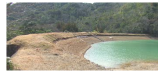
Eroded levee
