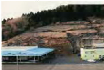
March 12: A slope collapsed just after the earthquake.
