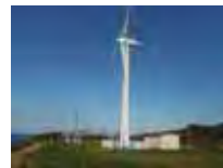
Tokuai Wind Power Station (Itoigawa City, Niigata Prefecture)
