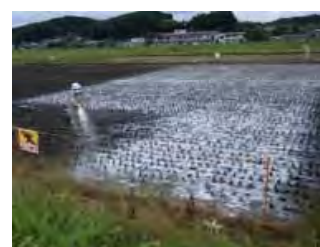
Using soil hardener for topsoil removal
