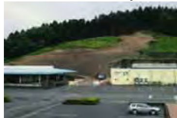
June 21: Filling cracks in emergency slope restoration
