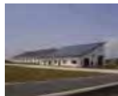
Solar panels installed on a compost facility (Sanmu City, Chiba Prefecture)
