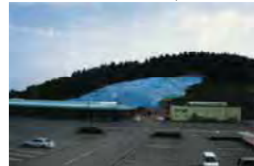
September 2: Laying blue sheets in emergency slope restoration
