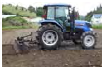
Basic topsoil removal
